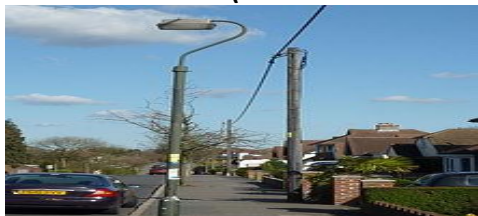
Figure 1: Example of an Insulated Bundle Electric Network
